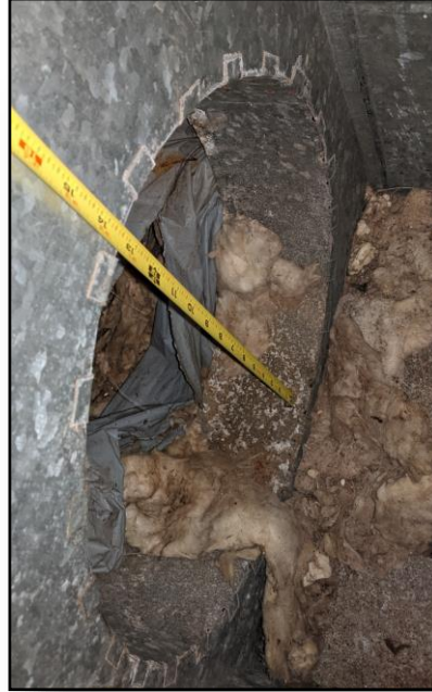
Disintegrated Outside Air Flex Duct
