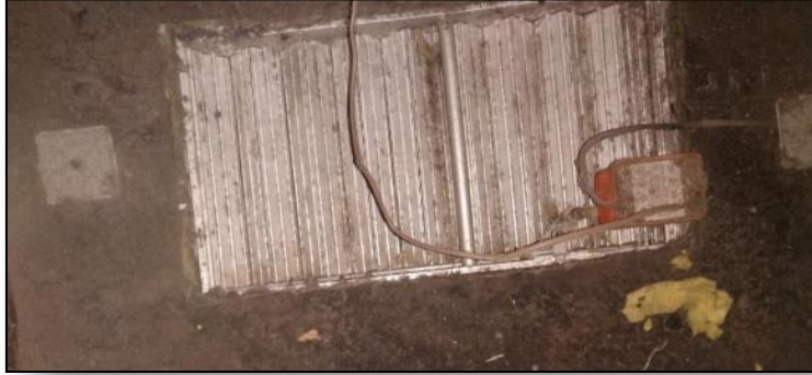
Broken Outside Air Damper
